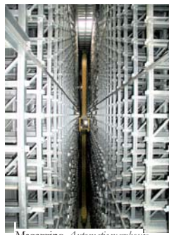
Magazzino Automatic warehouse
